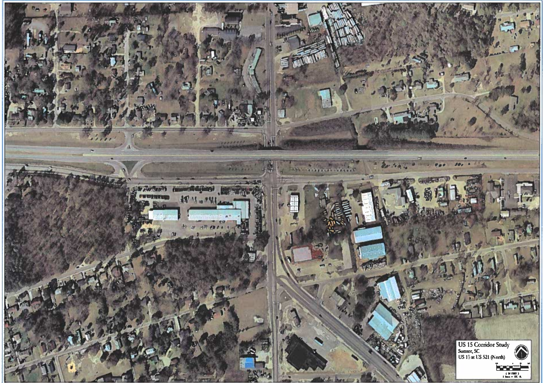
Lafayette Drive at US 378 Bypass – Existing Conditions
