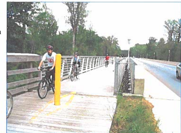
Example of Cantilever Pedestrian Bridge
