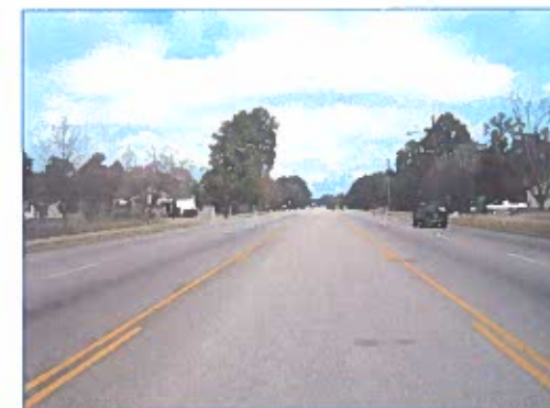
Existing typical section for most of Lafayette Drive
